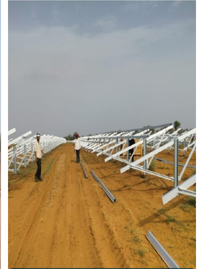
MMS rows going up
