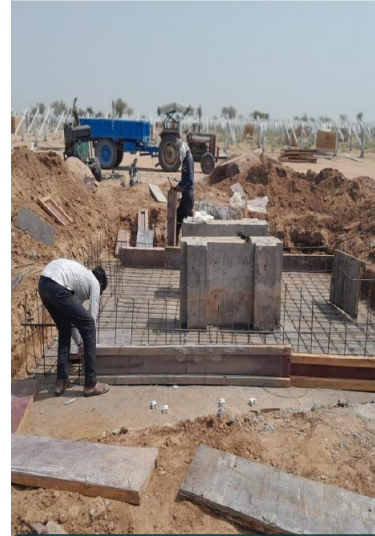
Foundation casting
