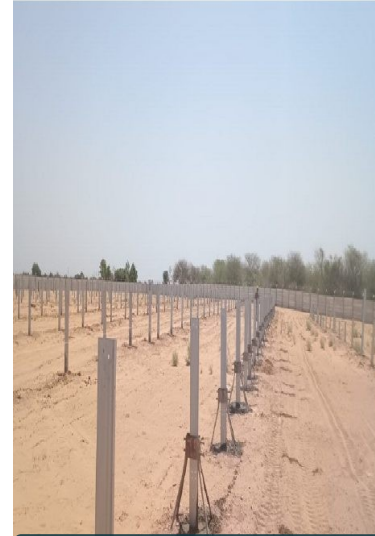
Column posts erected
